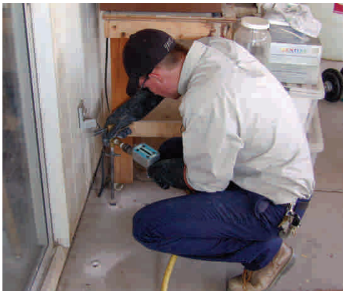
Figure 6. Application of termiticide into patio
